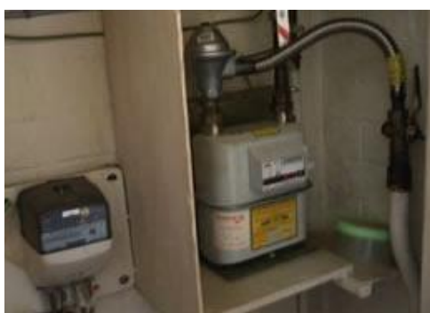
Asbestos panelling around a gas meter
