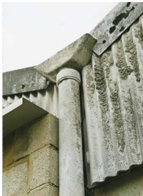
Asbestos cement downpipe, hopper and profile sheet
