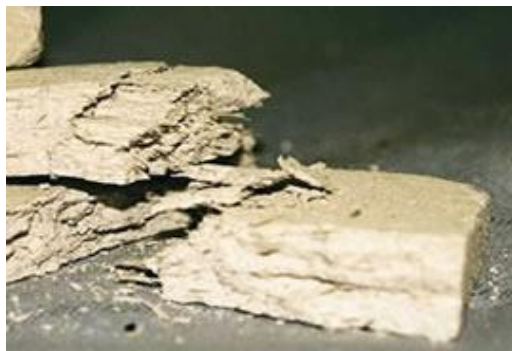
Pieces of Asbestos Insulating Board (AIB)
